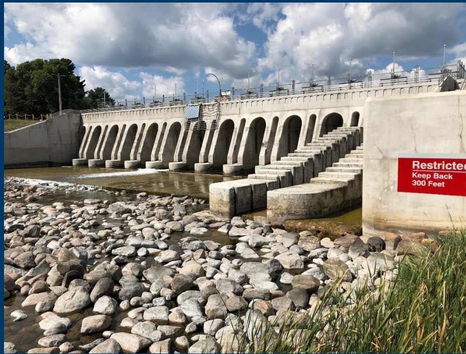
Pine River Dam at Cross Lake 8-29-21
